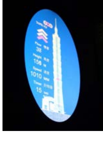
Fig. 1: Position and speed illustration in the lift of the Taipei 101 tower.
